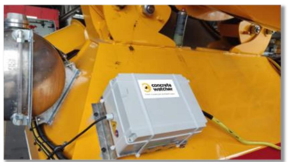
Fixing of the box with the electronics
